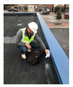
Look For The Following Damage – Common roof damage items to look out for include missing roofing material that may have blown off, debris, clogged drains, ponding water, damaged flashings, tears from debris or blistering/bubbling in your membrane caused by high winds and pressure changes, hail damage, interior leaks/water stains and moist insulation beneath the roof's surface.
