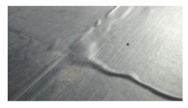
Blisters, bubbles, and cracks on the surface of the roof membrane are sure signs that it's time to replace the membrane.
