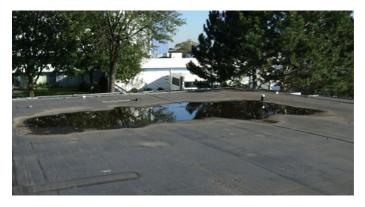
"Flat" roofs usually have at least a 15-degree slope to allow for water runoff, but as the roof ages, the roof could start to warp causing the designed runoff to become less effective and water to pool and puddle leading to increased water damage and leaks.
