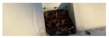
Some roofs have scuppers which are holes you can see from the outside of the building at the base of the roof's parapet walls. Because scuppers are slightly below the roof's surface, they can easily be clogged by dirt and cause standing water on the surface of your roof.
