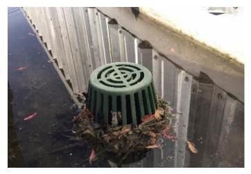
Clogged roof drains can cause standing water that will reduce the lifetime of your commercial roof. Just a small amount of pine needles or other tree debris can allow debris to penetrate and clog the drain pipes and cause standing water at the location of each clogged drain.
