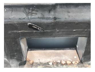
These deficiencies are typically caused by foot traffic, mechanical work, or loose debris on the roof.
