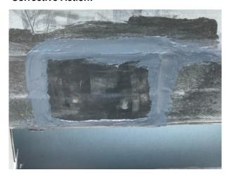
The area surrounding the deficiency was cleaned. A new piece of waterproofing membrane was installed and sealed per industry standards.
