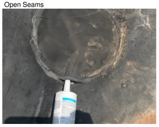
Open seams in the waterproofing membrane are typically caused by failing seam adhesives or membrane movement over time.
