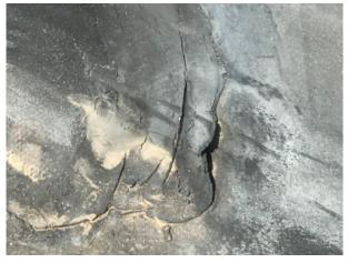
The existing caulk or sealant has failed due to age or improper application.
