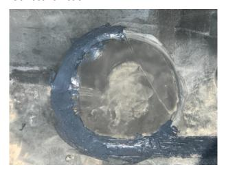
The area surrounding the open seam was cleaned and sealed per industry standards.
