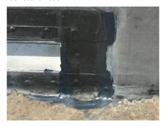
The old product was removed. The area was cleaned and new sealant installed as required to complete the repair.
